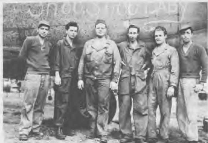
Sgt. Stoker's crew repairing damaged B-24 at Woodbridge emergency strip.
