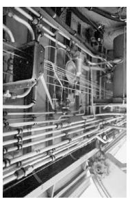
Looking toward tail, inside right bomb bay. Note complex and vulnerable rudder, aeleron and elevator control cables, hydraulic lines for flaps, landing gear, bomb bay doors, de-icer boots. Upper right corner shows part of wing spar. At lower right see roll-up bay door mechanism and open bomb bay.
