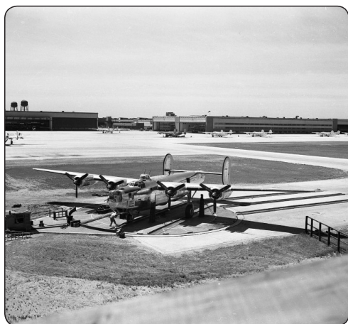
6-29-44: A FO B-24J at the “Compass Rose” where every ship was checked on a “non-magnetic” turntable.
