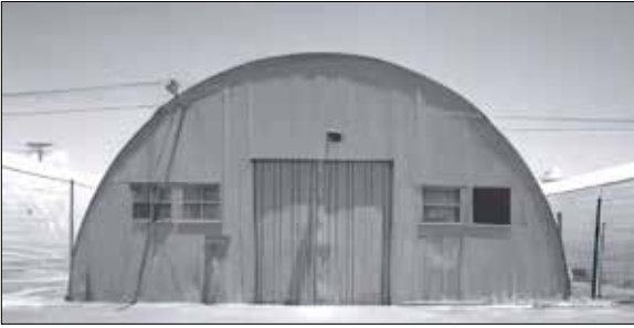
The difference in curvatures between a 392nd BG Nissen hut (top) and a Quonset hut (bottom) is the easiest way to tell them apart. Photos: Top: 392nd BG archives; Bottom: Wikipedia.
