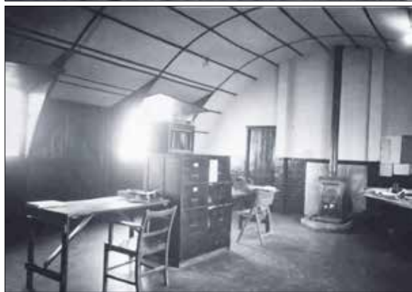
Top photo: Lt Col. Peter Nissen (left) and one of his huts in 1917. Middle: two 392nd Nissen huts. Bottom: the Station Orderly Section on 20 Feb 1945. The interior framing is clearly visible, as are dormer windows, doors at the back and side, and a stove. Photos: Top: Wikipedia. Middle & Bottom: 392nd BG archives.
