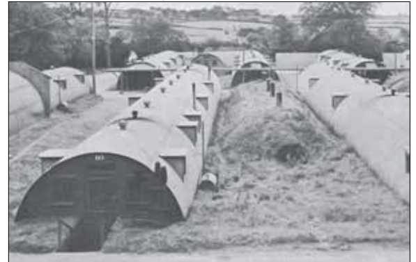
The above "Elephant Hut" was an enlarged version of the Quonset Hut, with dimensions of 40' x 100'. A construction team of ten men could build one shed in under 300 hours, an impressively small amount of manpower and time considering the building's size. It could also be shipped to any location in 23 crates and took up little room in a ship's cargo hold." This according to: http://quonset-hut.blogspot.com/p/morphology.html .
