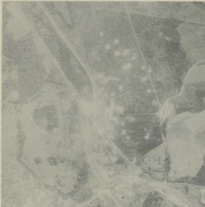
ANIZY R.R. BRIDGE: TINY TARGET Resistant to lighter-bomb attacks, steel cantilever bridge faces high altitude threat from 2000-pounders.
