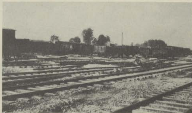
TRACKS STILL TWISTED AFTER REPAIR
